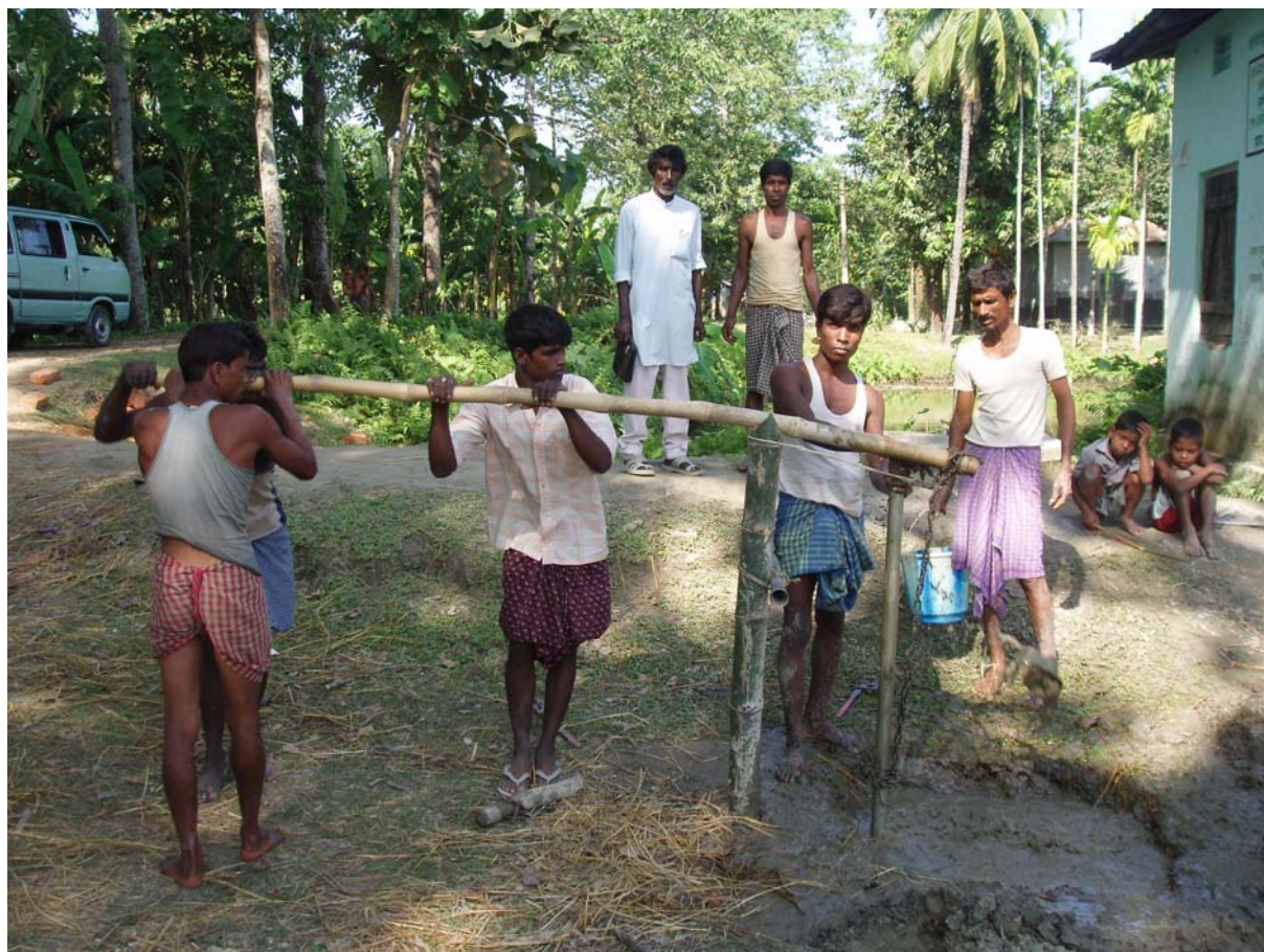
Figure 7. A group of drillers installing a tube well in a small village. Sediment samples were taken from the wells drilled during the time of the study.
